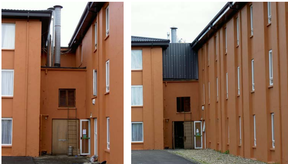
Figure 15: Pre-Installation Image Figure 16: Image after Installation
