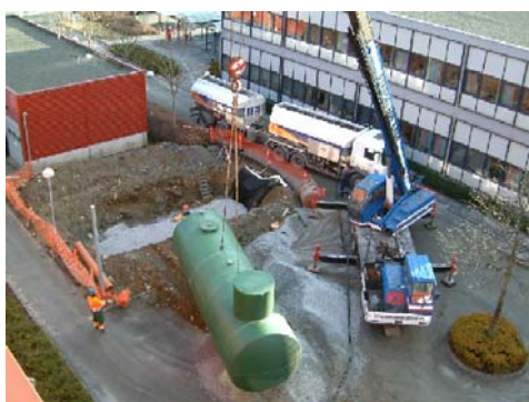
Figure 5: Installation of 30 m 3 Methanol Fuel Tank at Statoil Headquarters
