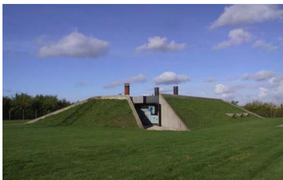
Figure 3: M/R-Station Lynge with Turbine Installed in Boiler Room
